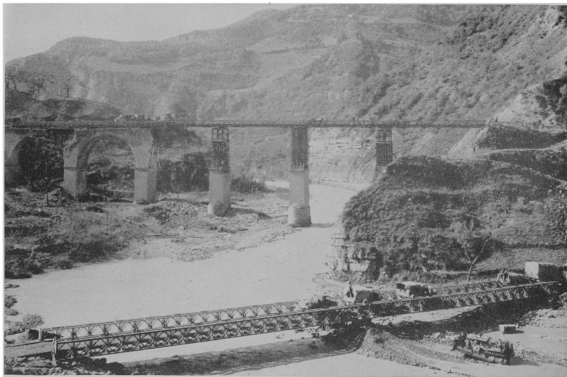
*Construction of this Bailey bridge eased supply problems for 13 Corps*
