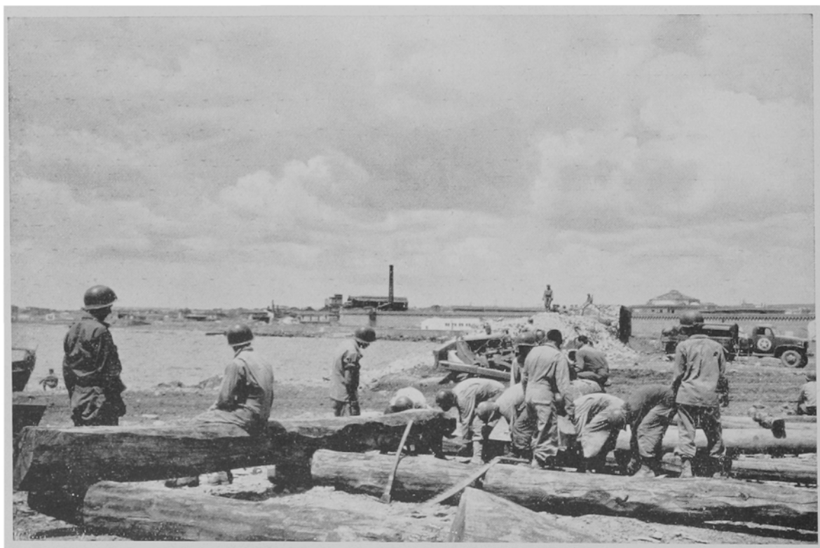
Fifth Army engineers at Civitavecchia prepare a wharf to unload ships.
