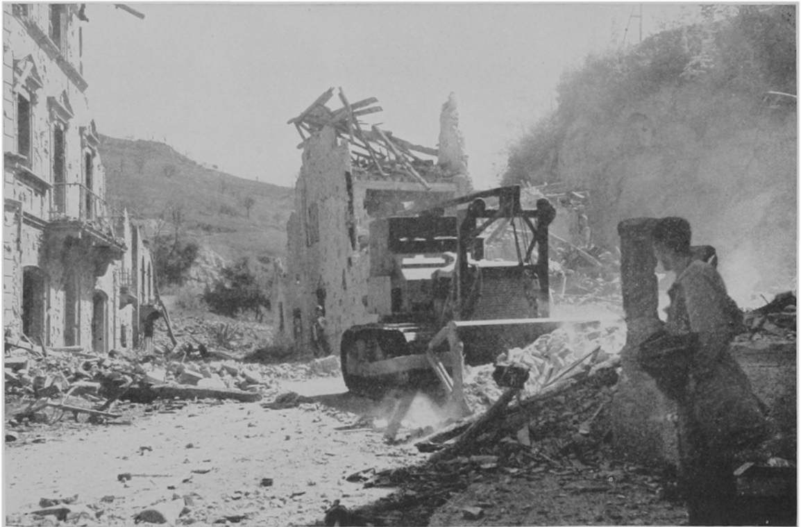
A bulldozer in Pianoro clears away the debris to open up Highway 65
