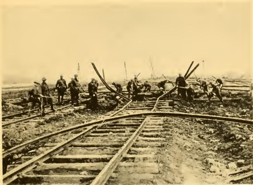
*View of destroyed railroad tracks at Waereghem, Belgium. These tracks were destroyed by mines before the Germans retreated from the city. Men working in picture are from Company A, 316th Engineers.*
