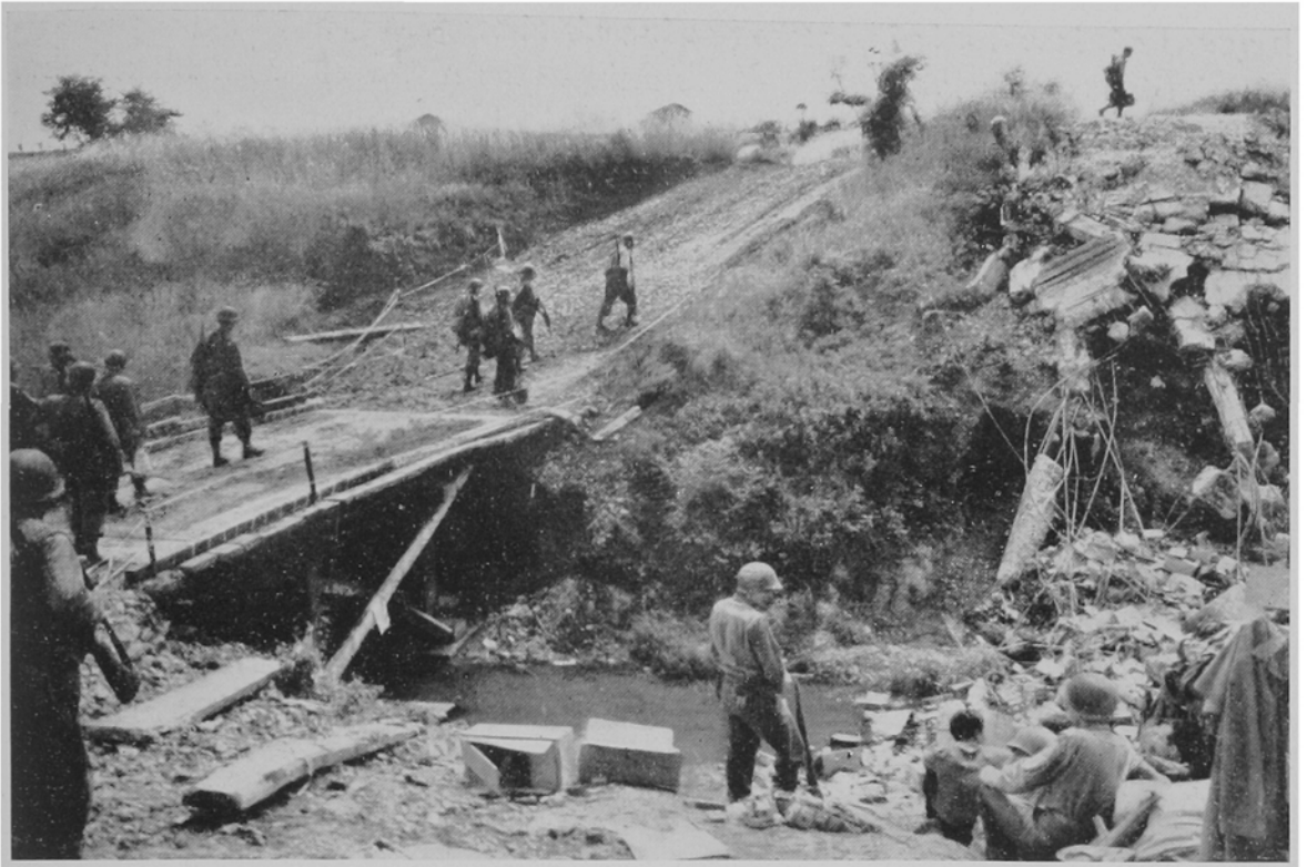
The engineers have completed a bridge which will further the advance.
