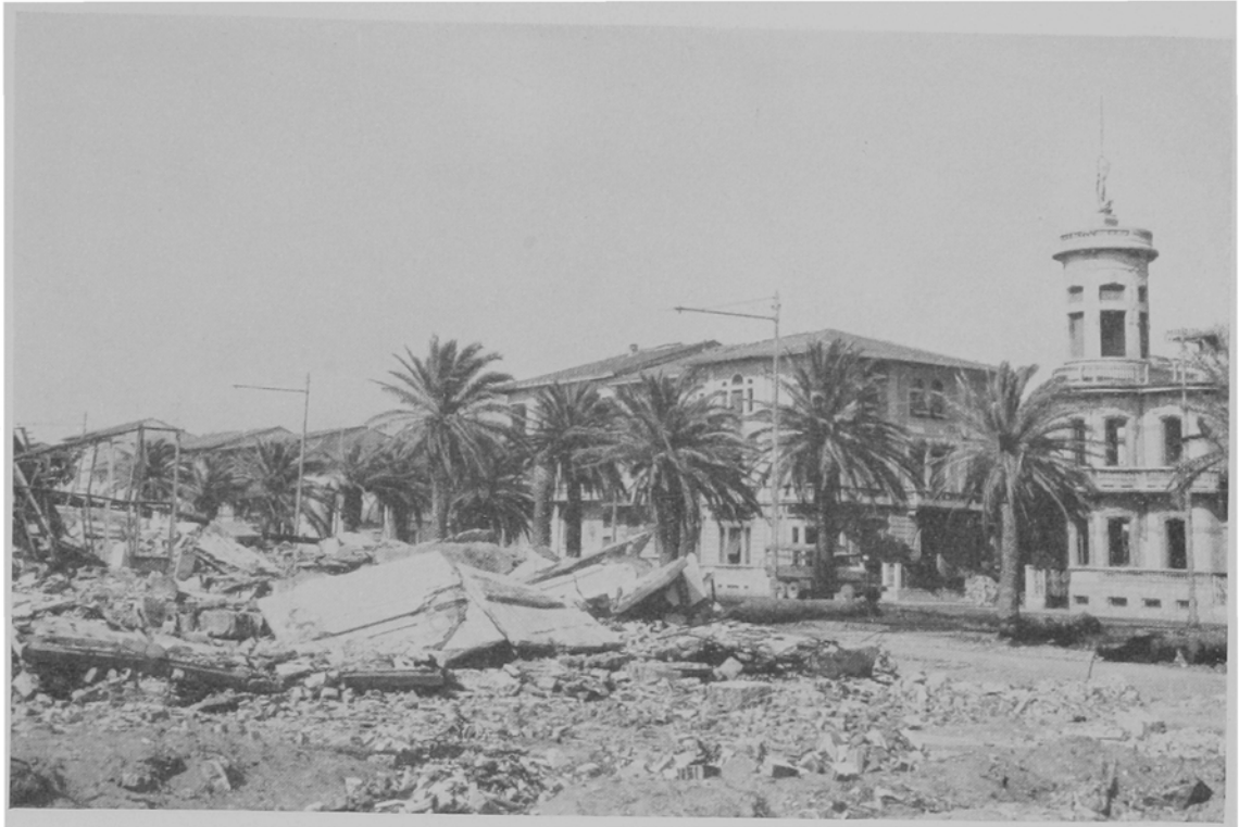
Troops of Task Force 45 found the resort town of Viareggio badly damaged
