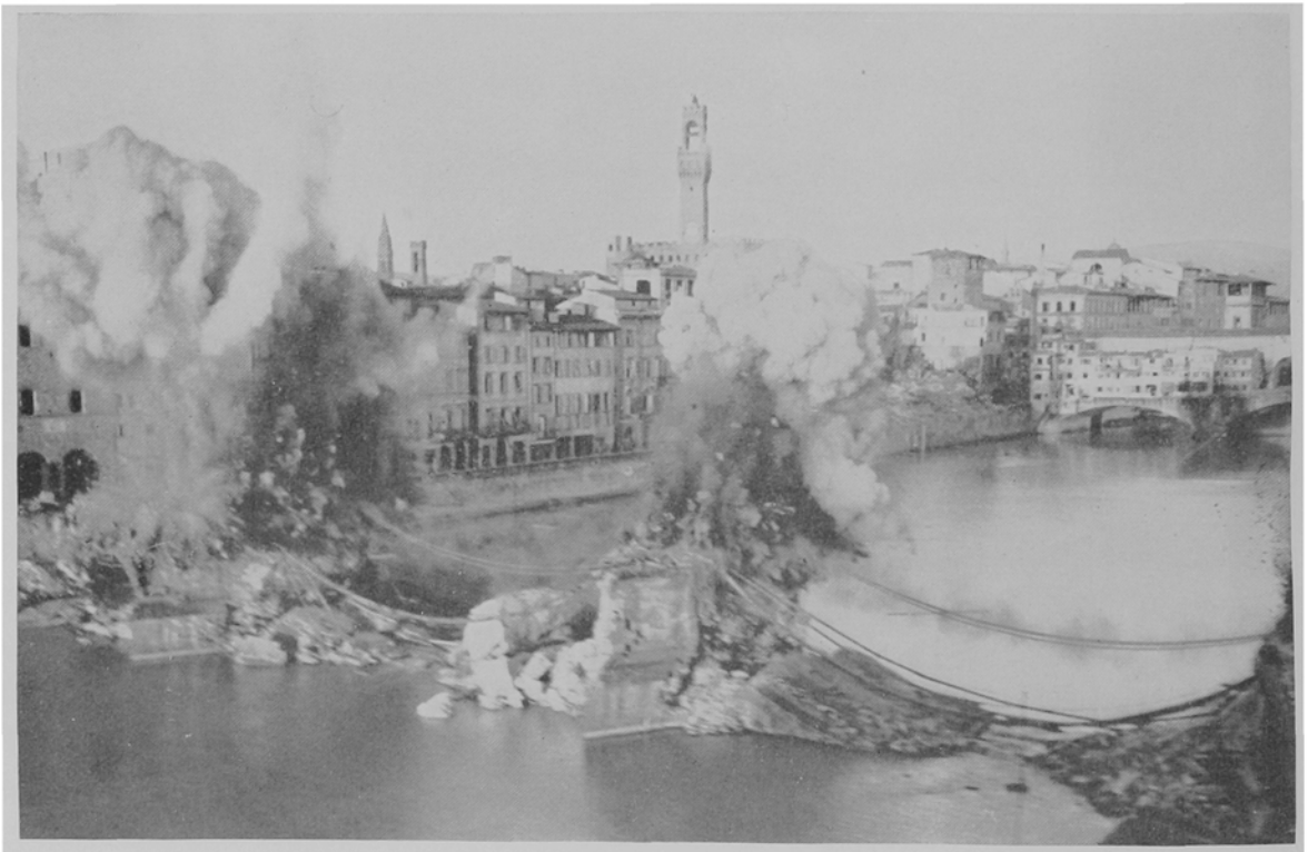
British engineers clear the way for a Bailey bridge across the Arno River
