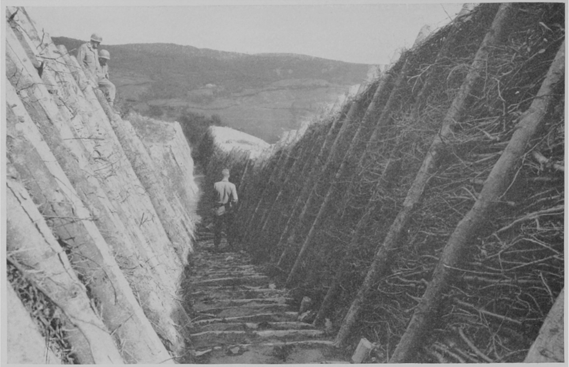
Antitank ditch constructed by the Todt Organization to protect Futa Pass
